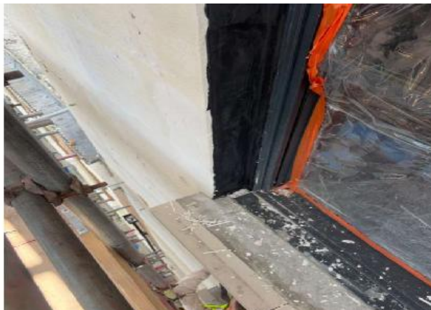
A photo Concrete repairs to stone work
