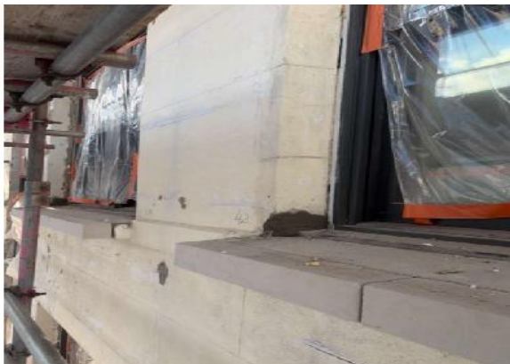
A photo Concrete repairs to stone work
