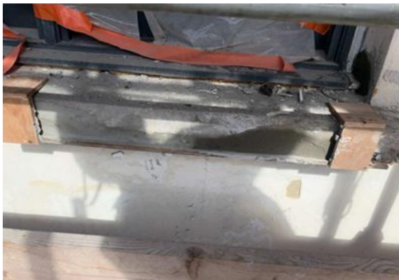
A photo Concrete repairs to stone work
